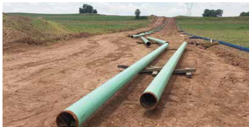
To construct a new pipeline, energy companies must navigate complex environmental regulations
